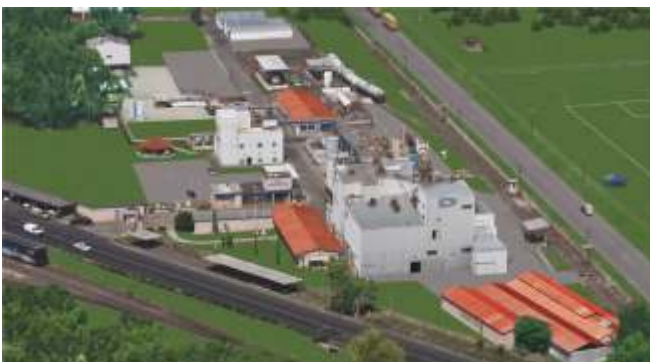
JRS plant Demacsa, Mexico
